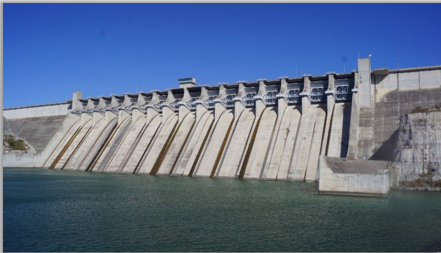
AMISTAD DAM DEL RIO, TEXAS
