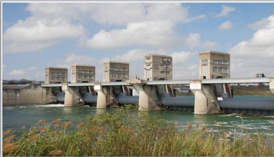
ANZALDUAS DAM HIDALGO COUNTY, TEXAS DSAC IV Low Urgency
