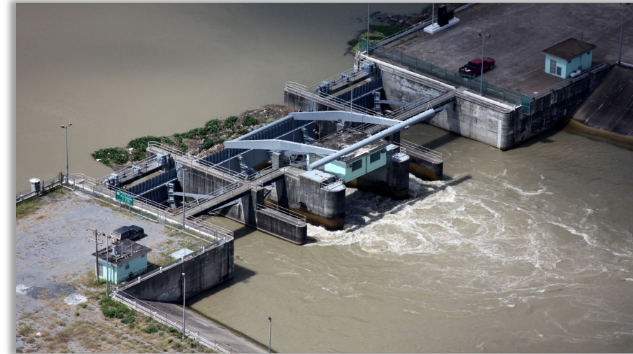
RETAMAL DAM HIDALGO COUNTY, TEXAS DSAC III Moderate Urgency
