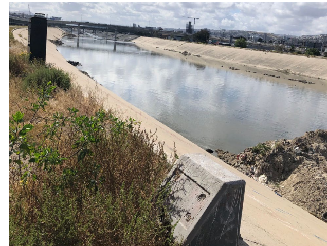
Tijuana River Levees – San Diego, CA
