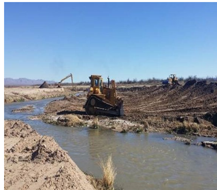
Removing sediment in El Paso, TX
