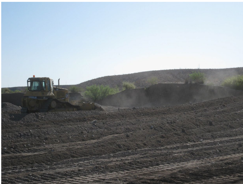
Removing sediment in Presidio, TX
