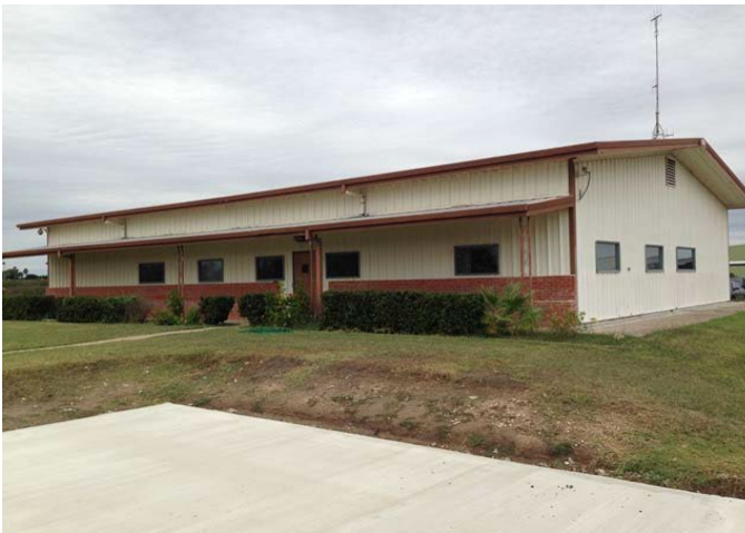
Admin Building – Mercedes, TX
