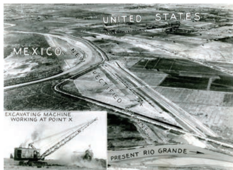
FIGURE 5: RECTIFICATION PROJECT, COURTESY USIBWC ARCHIVES.
