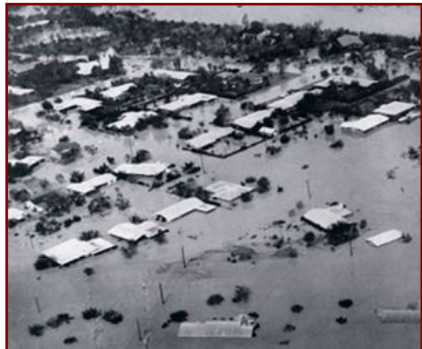
Hurricane Beulah Flooding
