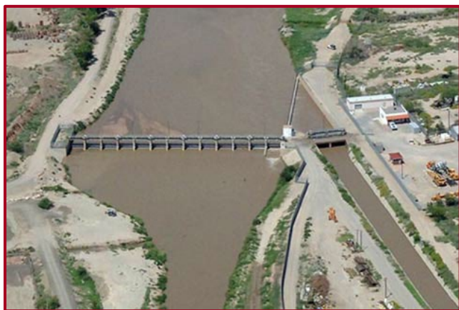
American Diversion Dam
