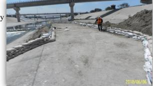
Construction of the sandbag weir in the Tijuana River channel in Mexico.
