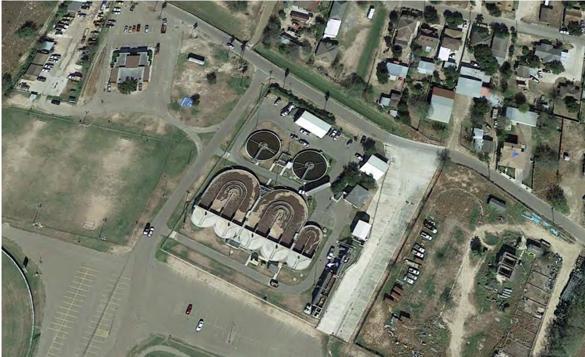
The City of Roma's Wastewater Treatment Facility
