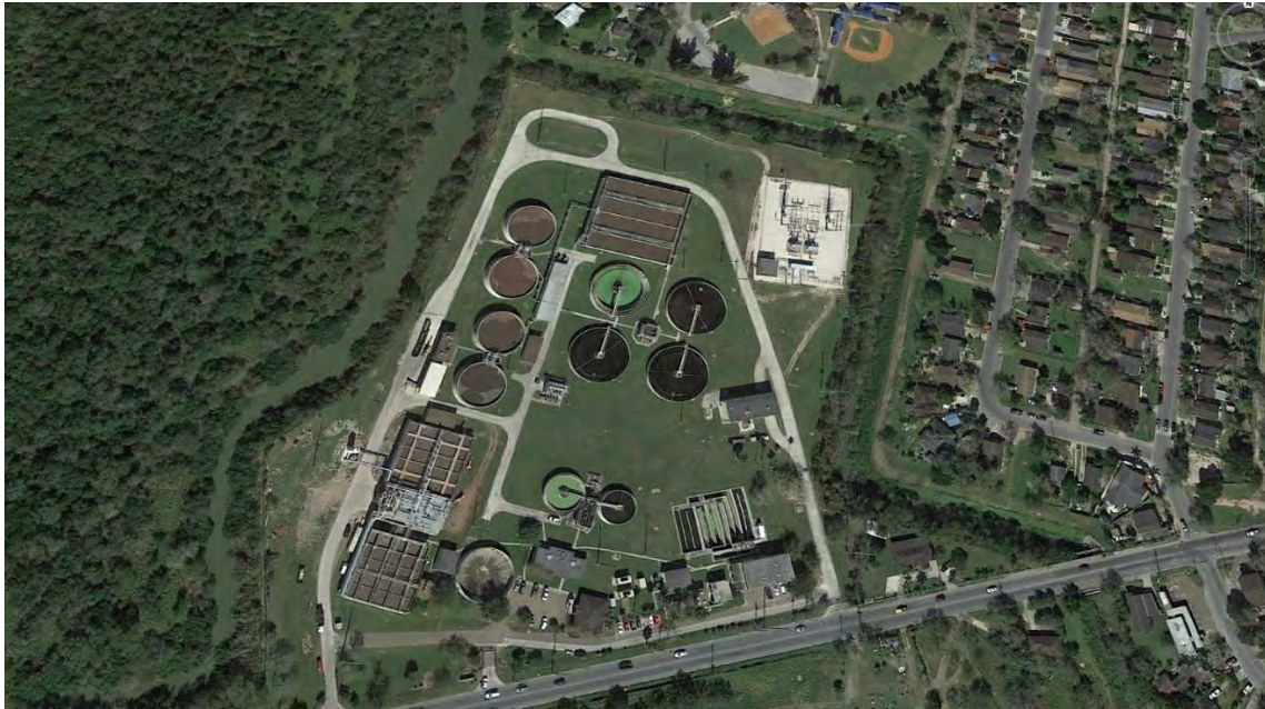
The Brownsville PUB's Southside Wastewater Treatment Facility
