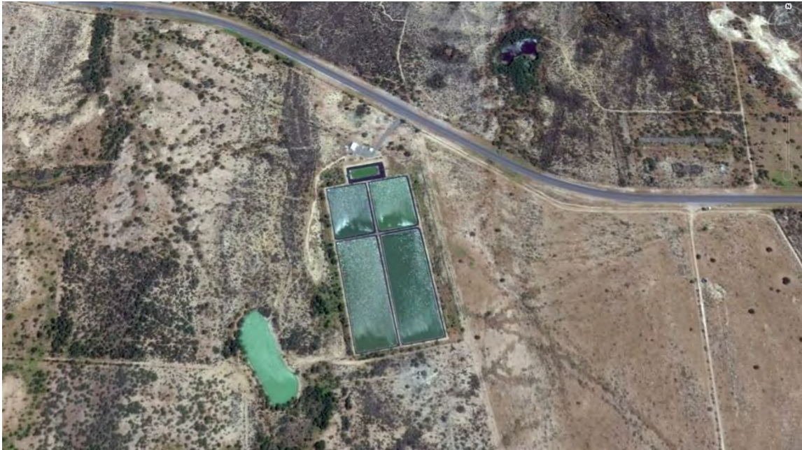
Ciudad Mier's Wastewater Treatment Facility
