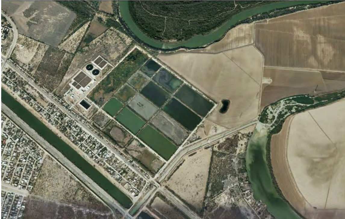
The City of Reynosa Wastewater Treatment Facility No. 1 (PTAR No. 1)
