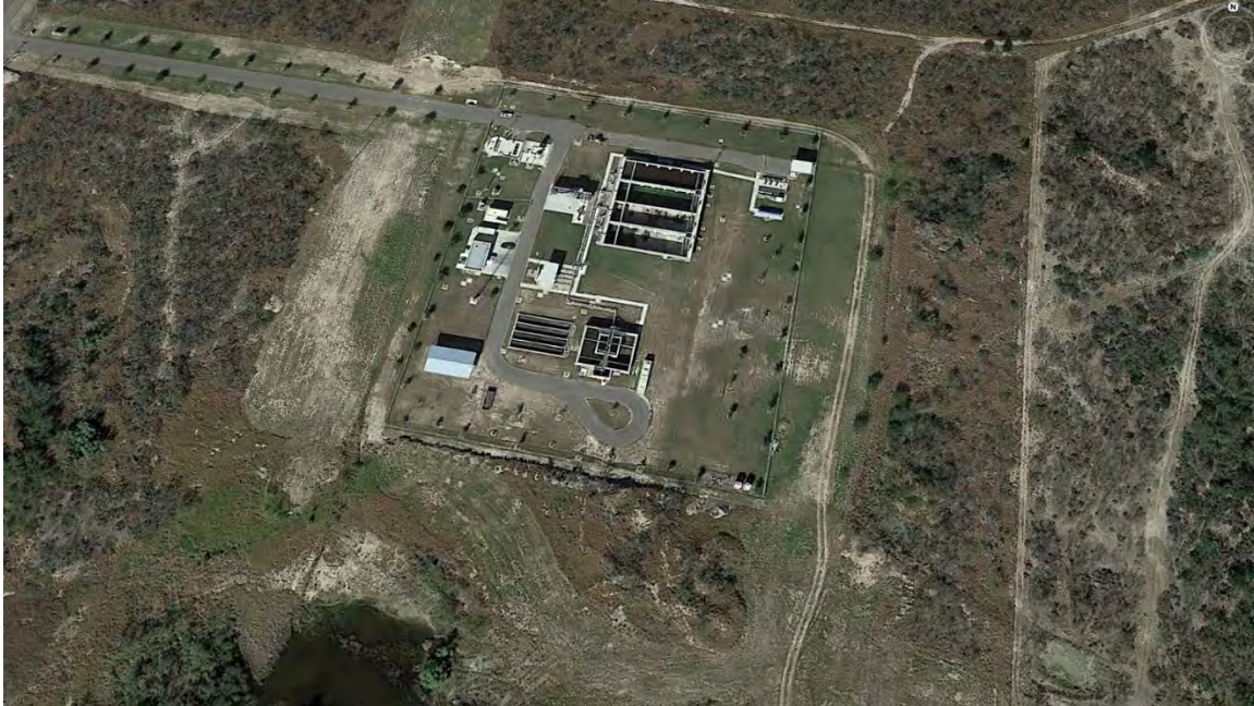
The AGUA Special Utility District's Wastewater Treatment Facility
