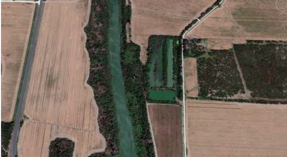
Ciudad Camargo's Wastewater Treatment Facility
