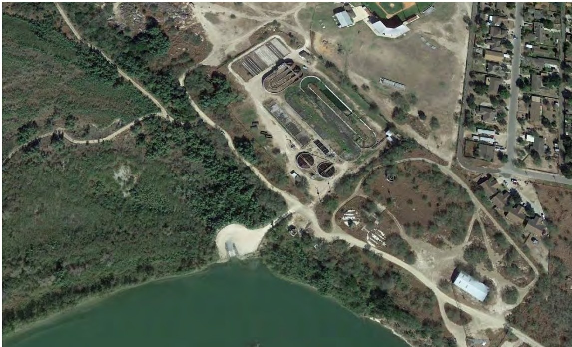
The City of Rio Grande City's Wastewater Treatment Facility
