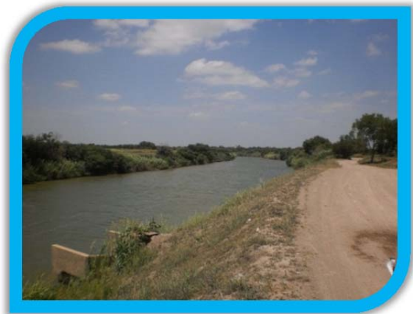
El Jardin Pump Station Facing Upstream at Station 13177 in Assessment Unit 2302_01
