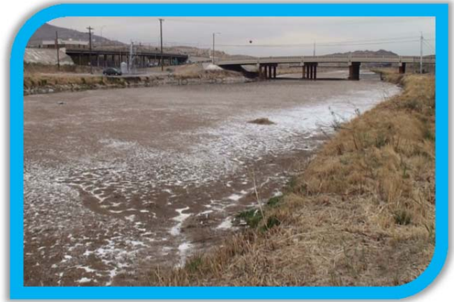
Salt Deposits from Water Evaporation at the Courchesne Bridge in El Paso, Texas
