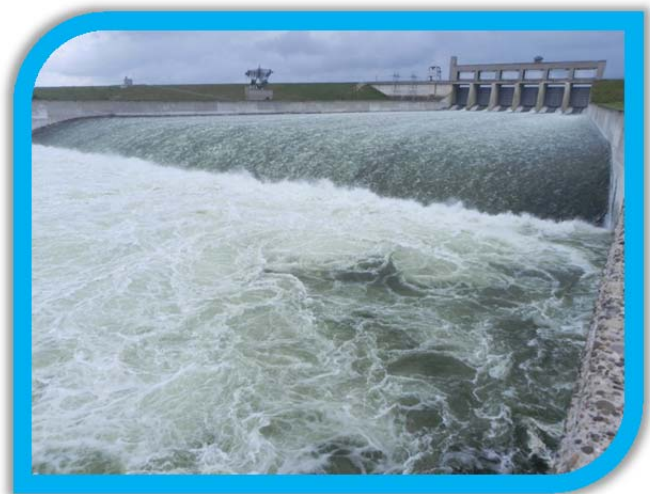
International Falcon Dam Release of Floodwaters after Hurricane Alex in 2010
