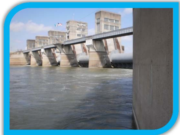
International Falcon Reservoir at Dam Assessment Unit 2303_03
