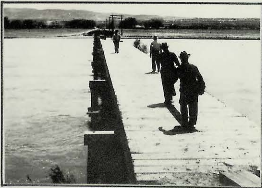
SALEM BRIDGE - Dona Ana County crew at work
