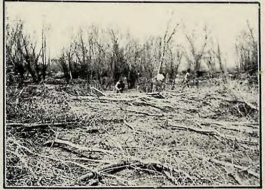
Clearing right of way by hand
