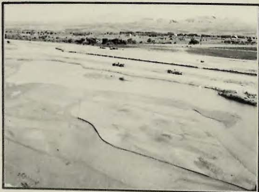
Channel Cut-off near Hill, N. M.
