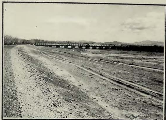
Looking downstream at Santo Tomas Bridge
