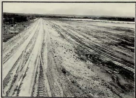
Looking downstream from Station 650 - Feature 301
