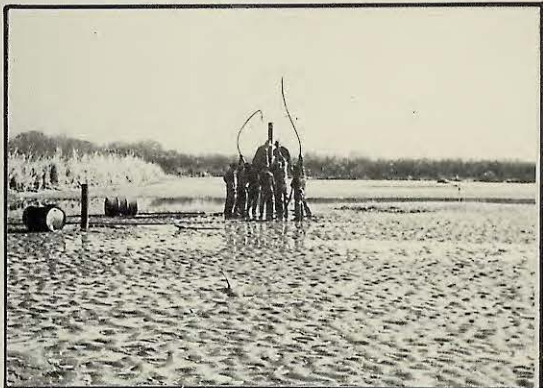
Crew jetting piling
