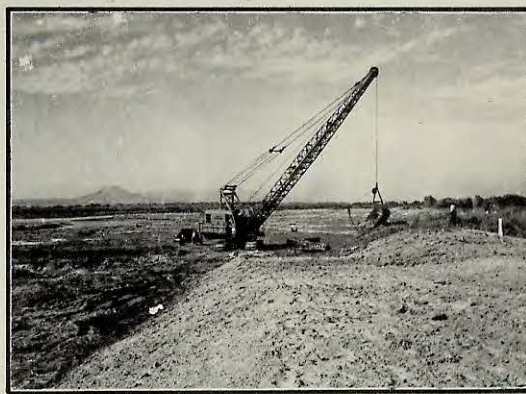
DRAGLINE No. 9 - Building levee
