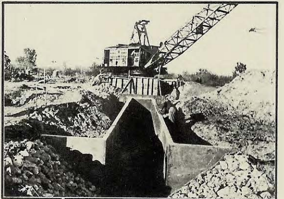
Brazito Lateral Wasteway
