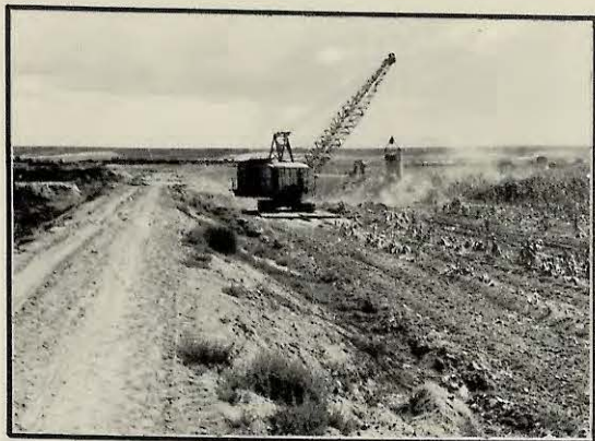
DRAGLINE No. 3 - Building levee
