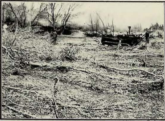
Clearing right of way with tractor
