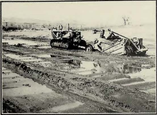
Carryall excavating low flow channel - Rincon Valley
