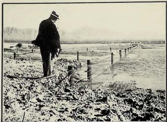
Revetment on East Levee near Vinton Bridge
