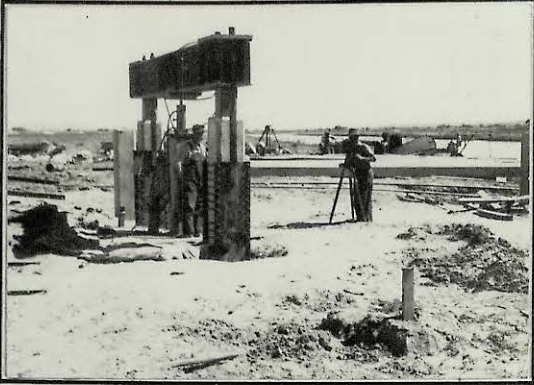
Testing concrete piles
