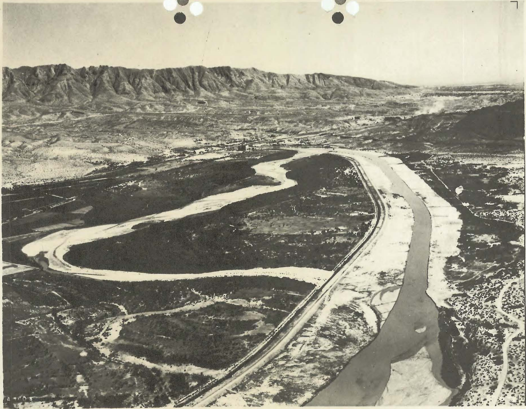
Downstream View of Jundt Cut-off
