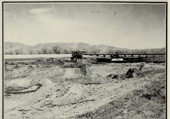
Tractor filling pit near Santo Tomas Bridge - Mesilla Valley
