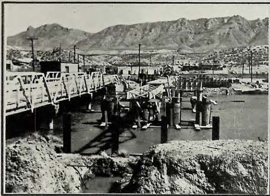
COURCHESNE BRIDGE - Construction of new concrete bridge
