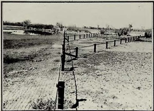
Revetment on East Levee Station 850 - Feature 401
