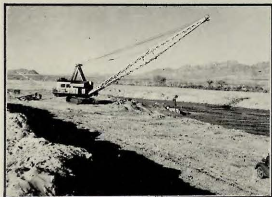
DRAGLINE No. 5 - Excavating Mesquite Cut-off
