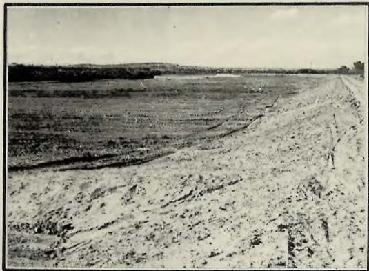
Completed levee and channel near El Paso
