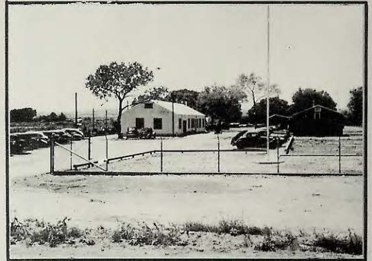
Warehouse and yard - Hatch
