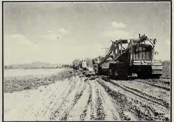
Carryalls plating levee - Mesilla Valley
