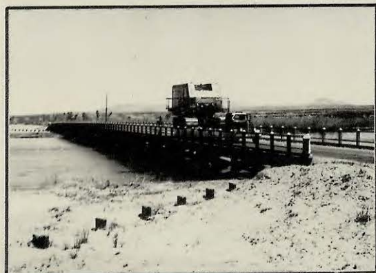
DRAGLINE No. 8 - Being moved across Hatch Highway Bridge
