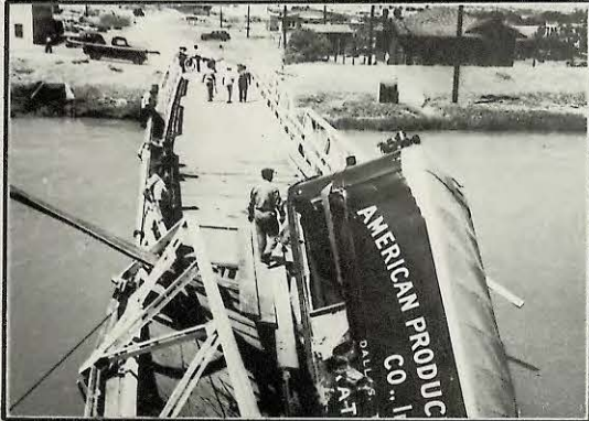
COURCHESNE BRIDGE - Heavily loaded truck breaks through bridge
