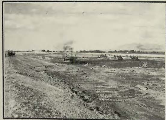
Tractors filling borrow pits - Mesilla Valley
