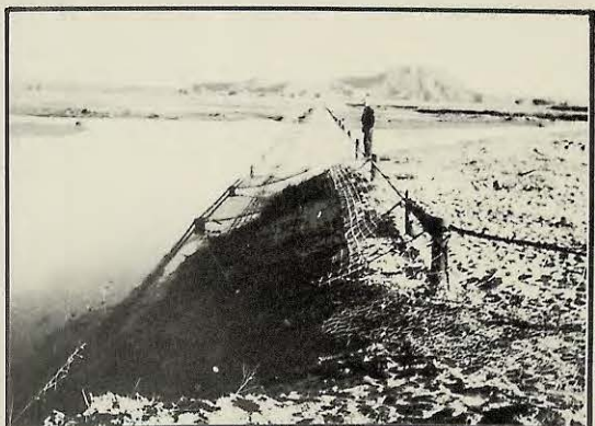
Special type of revetment - Rincon Valley
