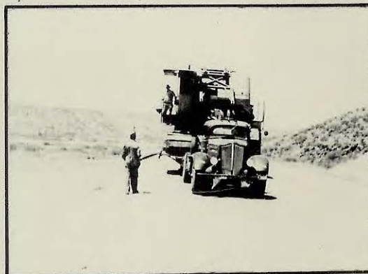
DRAGLINE No. 8 - Being hauled from Hatch to Las Cruces
