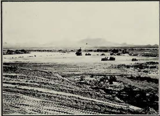
View of excavation equipment working - Mesilla Valley
