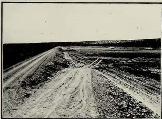
Looking downstream from Station 1090 - Feature 301
