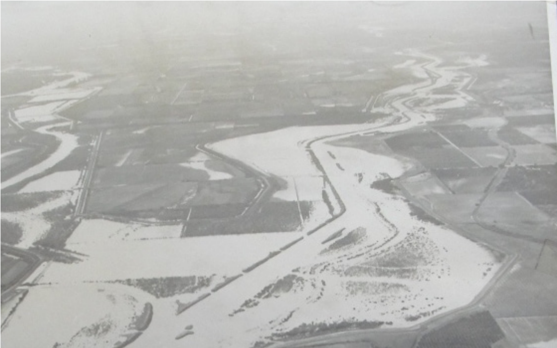
September 14, 1948: Looking west over the Mission Branch and Hackney Lake Branch floodways at their junction with the Main Floodway, with the Pharr south highway crossing the Main Floodway in the foreground. River overflow in the floodways, near maximum for this this flood at the time of the photograph, reached 6,040 second feet in the Mission Branch and 11,735 second feet in the Hackney Lake Branch.
