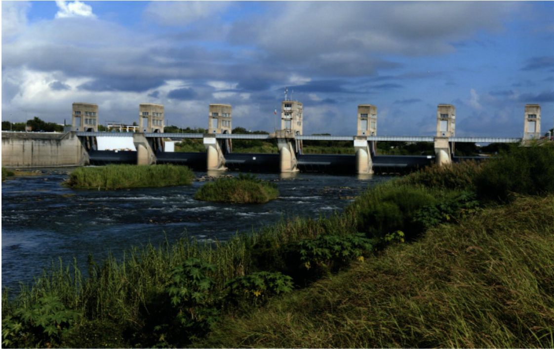
Pictured: Anzalduas Dam, near McAllen, TX
