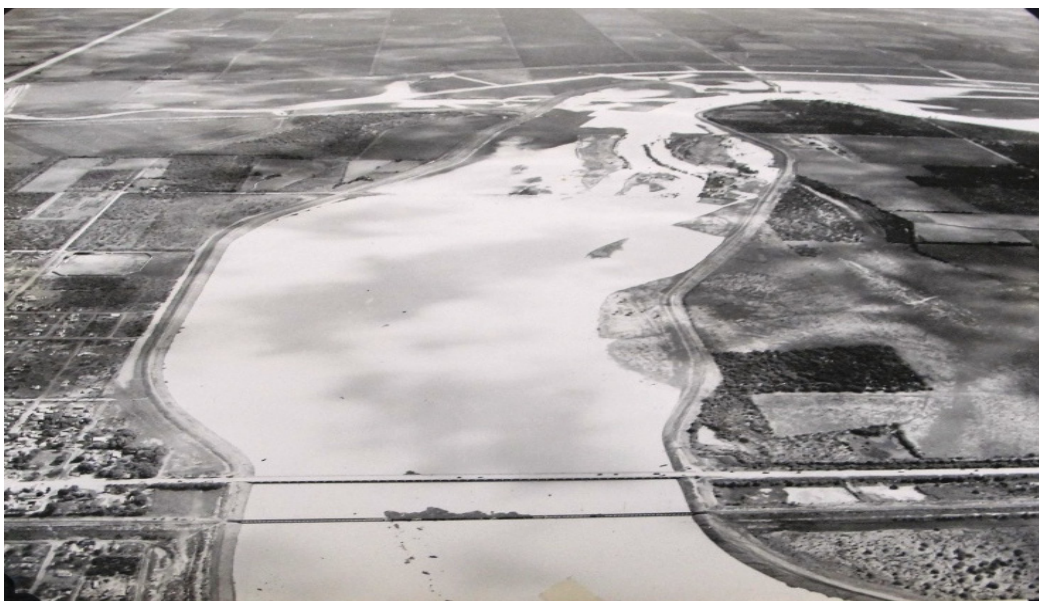
September 16, 1948: Looking south over the upstream end of the North Floodway from a point north of the highway and railroad bridges at Mercedes, TX. The junction of the floodway with the Main and Arroyo Colorado Floodways in visible in the background. Flow in the North Floodway during the mid-September flood reached a maximum at this point of 13,000 second feet the day before and was near maximum at the time of this photo.
