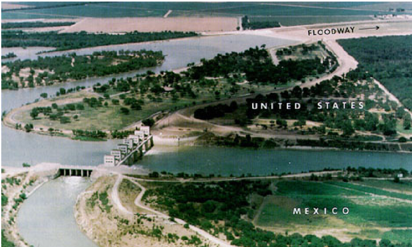
Early Aerial Photograph of Anzalduas Diversion Dam near Mission, Texas on the Rio Grande showing the U.S. off-river “Banker” Floodway, which, as a principle part of the International Project for control of floods of the Lower Rio Grande, serves to divert floodwaters from the river to the U.S. floodways. This photo also shows Mexico’s intake structure to its Anzalduas Irrigation Canal.
