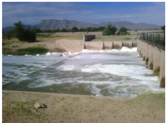
Rio Grande at Alamo grade control structure
