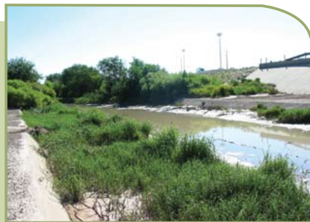
Figure 23 Concrete lined section of Rio Grande in segment 2308
