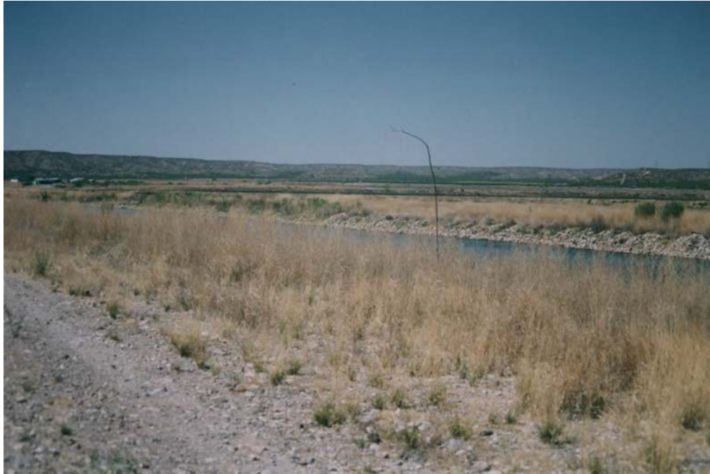
G1: Armored river bank. Wide flood plain dominated by sand dropseed. Several dead pole plantings.
