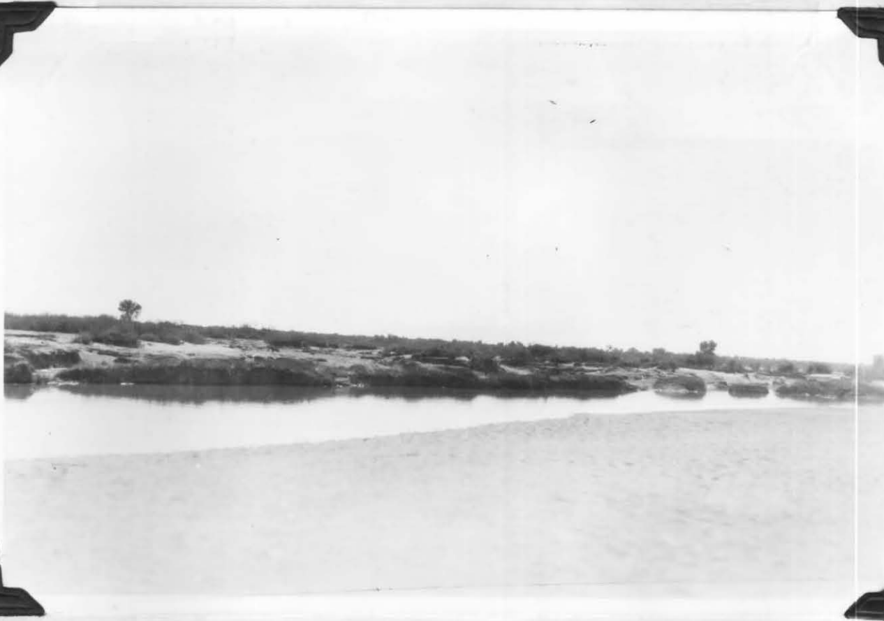
Scouring of ground on left bank of Rio Grande at entrance of Tornillo diversion canal.
