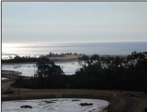
Lagoons at SABWWTP
