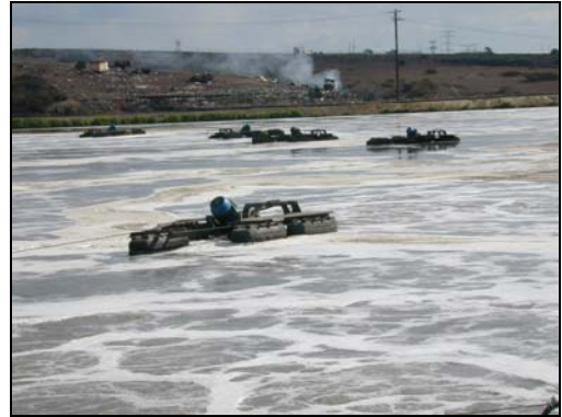
Aeration Lagoon at SABWWTP (Pond 1)
