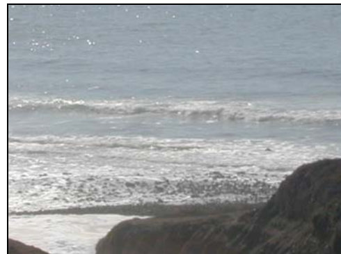
Ocean Discharge from SABWWTP
