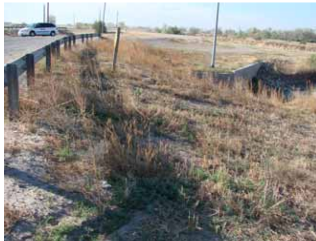
Facing downstream, guardrail discharge from RGACE to Rio Grande.
