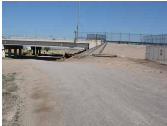
Levee at Ysleta Bridge, looking upstream
