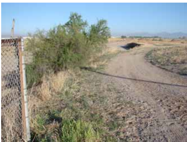
Levee system looking upstream from the Riverside headgates.
