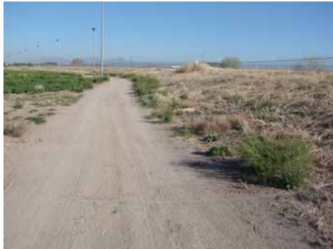
Levee toe is at Border Patrol access road. Light poles are 19 feet from levee toe.
