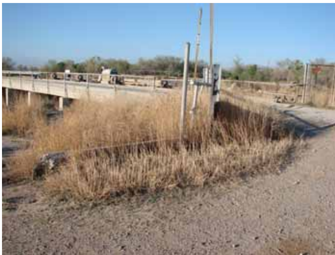
Bridge at diversion gates.
