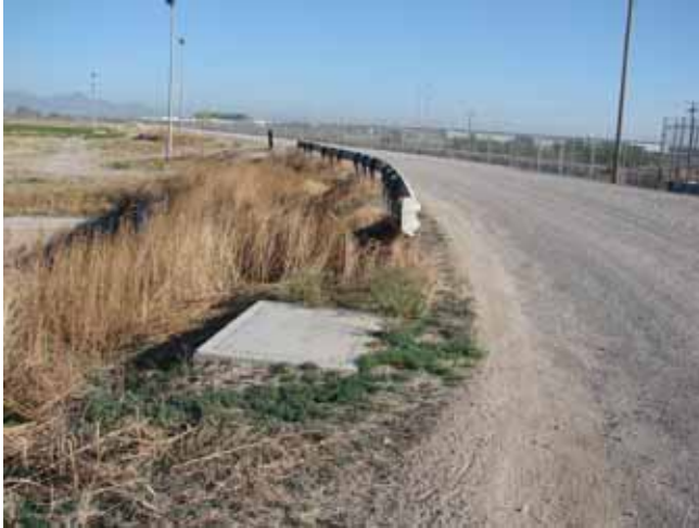
Guardrail at RGACE, facing upstream of Riverside Dam.
