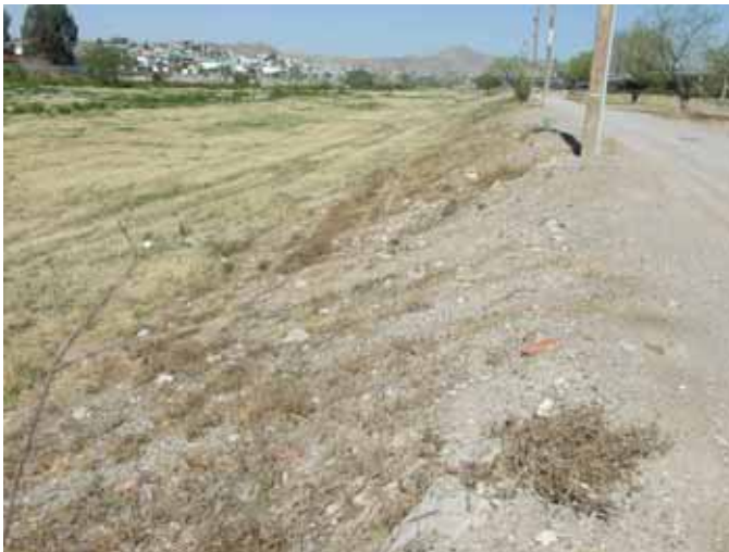
Downstream view of levee.
