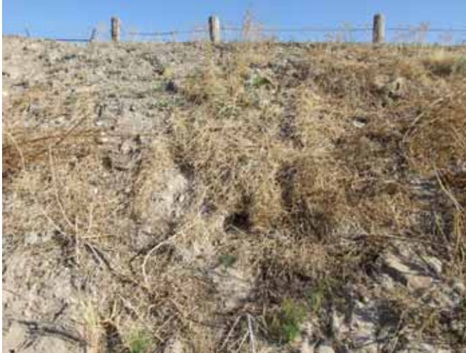
Photo of survey point looking up to the top of levee.
