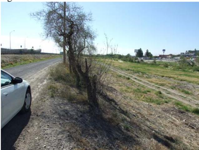
Photo showing 24 foot expansion footprint. The levee would now only be extended six feet only reaching the first patch of brush on the bottom center of this photo.
