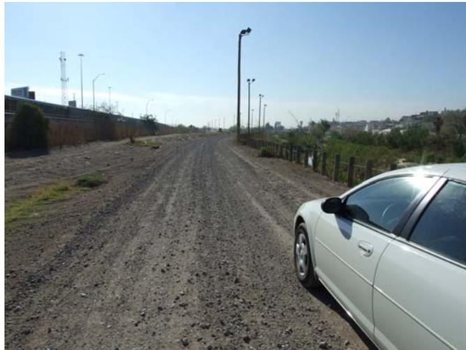
Erosion that is occurring in portions of the levee in this section.
