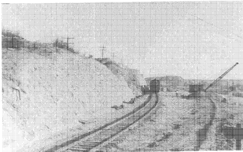
Plate 25. Relocation of AT&SF Railway Tracks, 19 October 1937.
