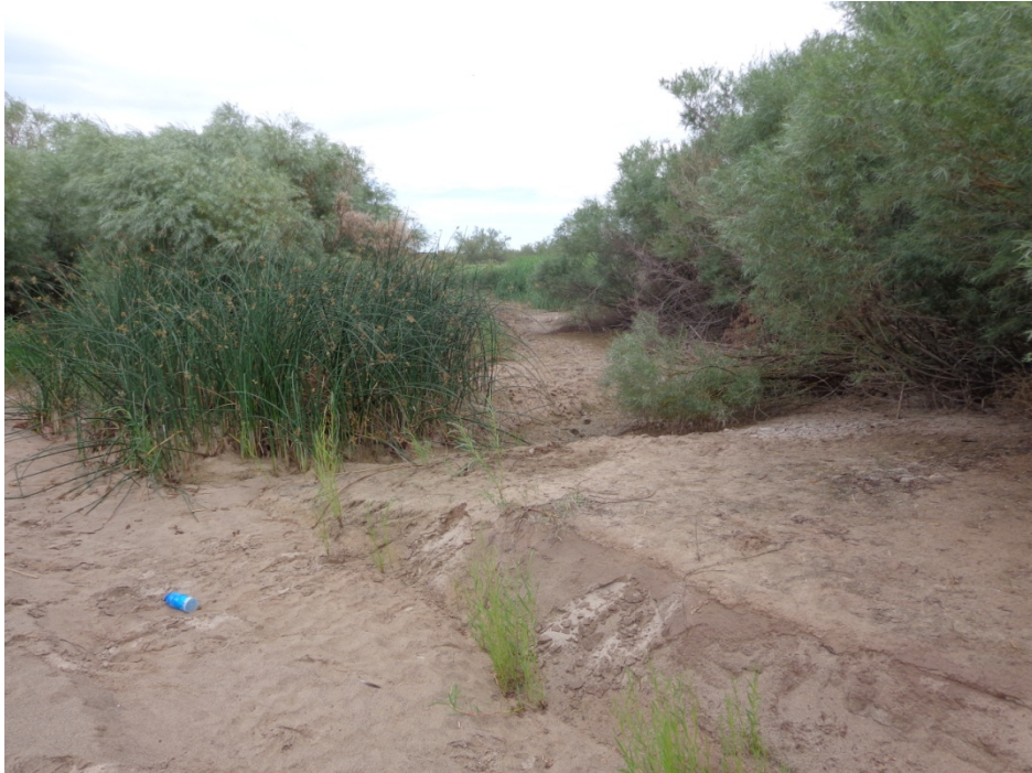
Confluence of Del Rio Drain and Rio Grande, will be extended to meet new alignment
